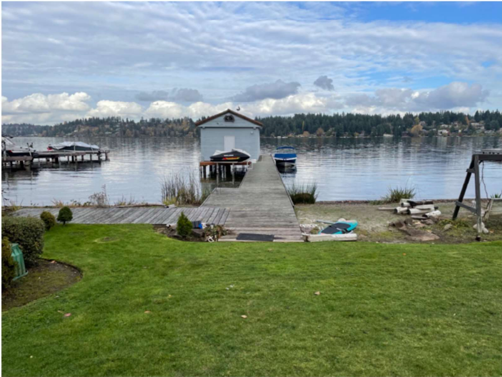
Photo 1 - Existing dock looking waterward.
