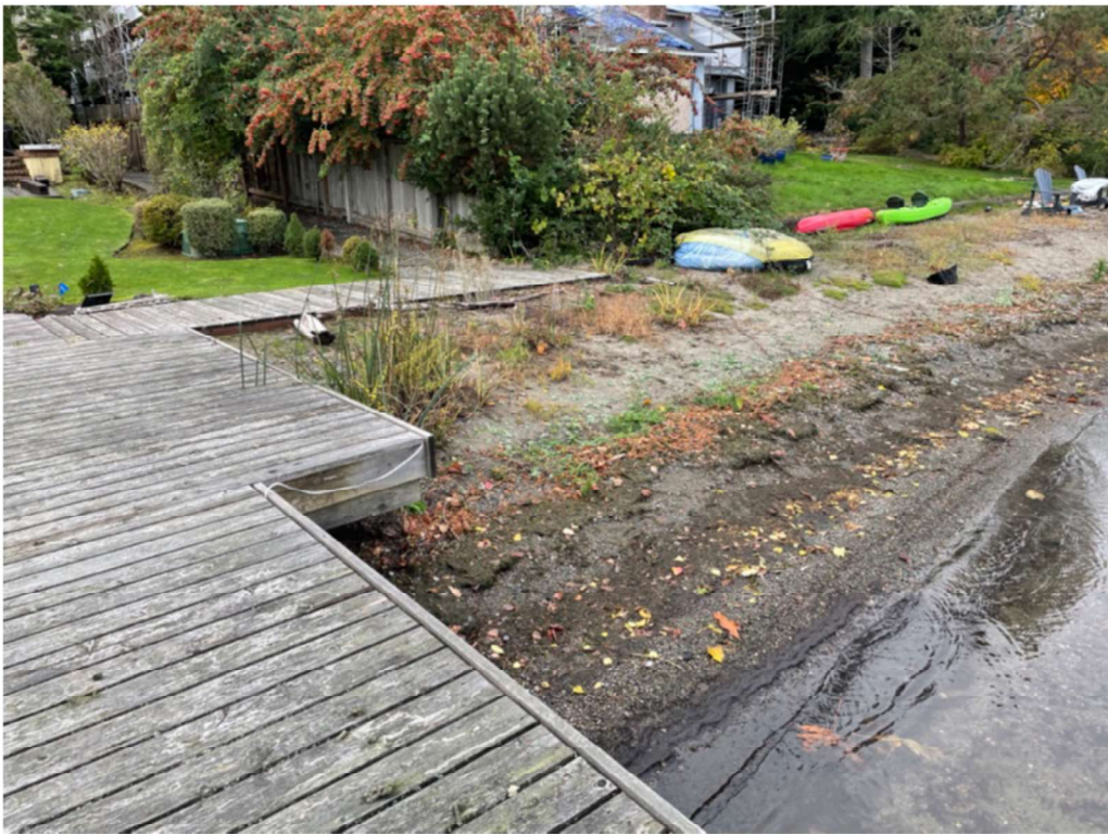
Photo 4 - Shoreline conditions looking West.
